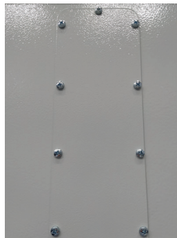
Fig. 8 Blind flange for the connection to the power supply (view from the bottom of the electrical cabinet)
