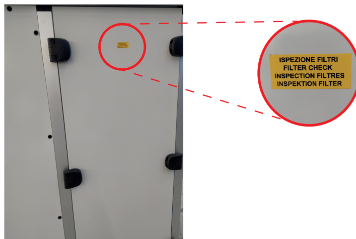
Fig. 26 Panel giving access to filters
